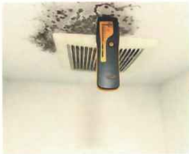
Normal Moisture Content - Master Bath
