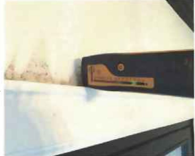
Normal Moisture Content - Exterior Door Trim
