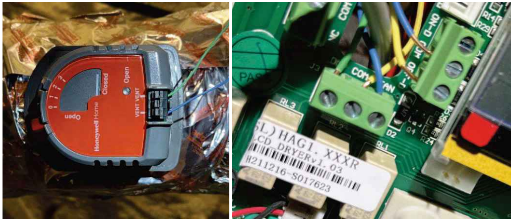
Figure 2: The fresh air damper on the right is using the green and blue wires; these are wired to the DMP and FAN terminals on the DE3000R controller, effectively disabling the fresh air damper.
