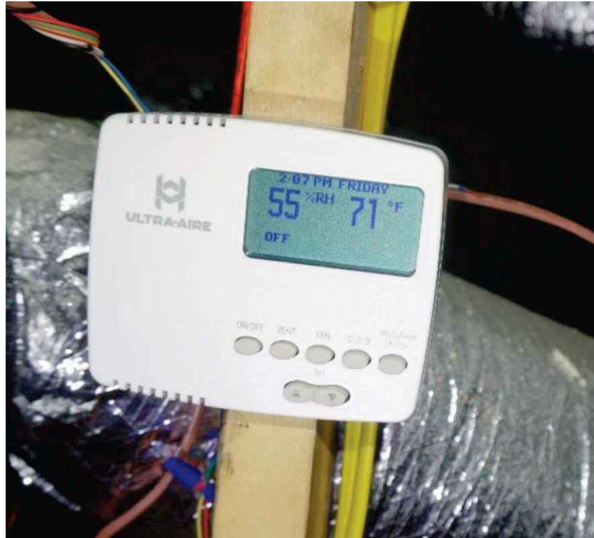
Figure 10: This photo excerpt from the 2025 CDC report shows that the dehumidifier has been turned off. This was confirmed in the text of the CDC report.
