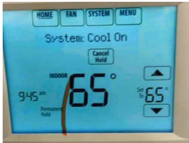
Figure 9: A photograph, ostensibly from the homeowner and dated 5/31/2024, showing the thermostat set to (and holding) a permanent temperature setting of 65°F.
