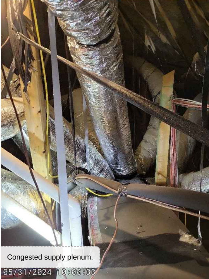
Missing insulation on refrigerant line in attic.
